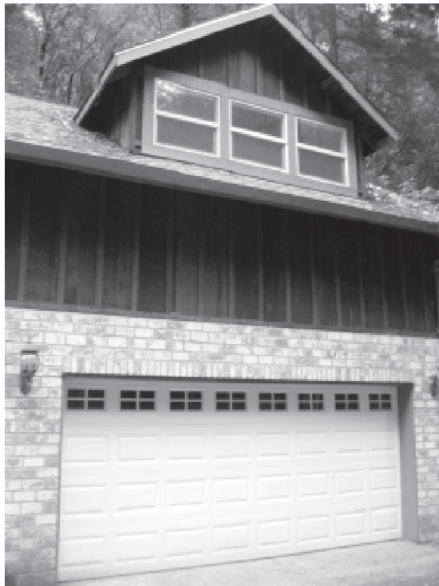
MAPS' new two-story office at Love Creek has a "shipping facility" on ground level with a spacious office and meeting room upstairs.
